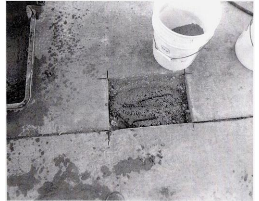
Add 1 Gallon of water per 50 LB bag of KF-K and mix thoroughly.
